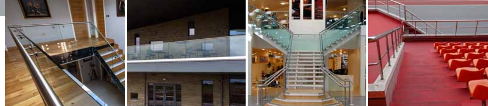
INTERNAL HOUSING 0.36KN EXTERNAL HOUSING 0.74KN OFFICE FUNCTION 0.74KN PUBLIC AREAS 1.5KN STADIUM FUNCTION 3.0KN
